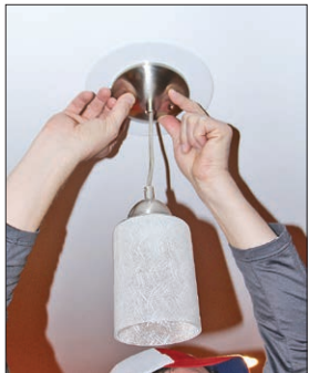
Wire & install new pendant fixture.
