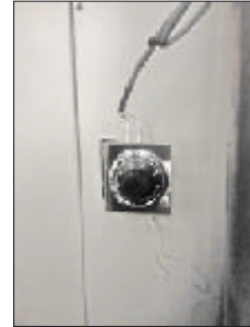
Humidifier safety thermostat
