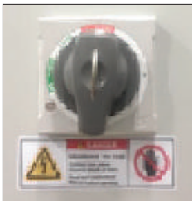
Figure 5-0 SEC 4100 - Main Power Switch
