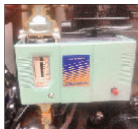
Compressor oil low switch
