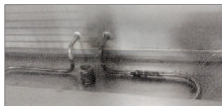
Humidifier Pan and Heating Coil
