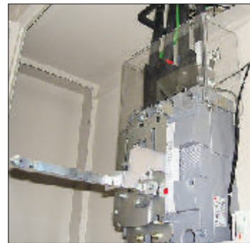
Figure 3-1 AC Supply Connections - SEC 4100
