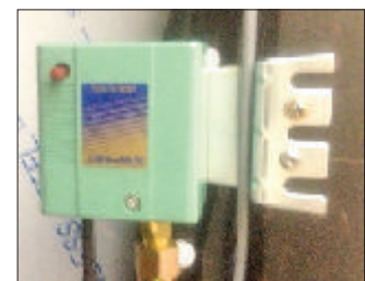
Compressor refrigerant high pressure switch
