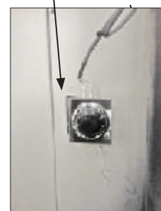
Safety Thermostat Humidifier
