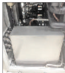
Humidifier DI Water Tank and Float Valve
