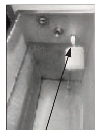
Humidifier DI Water Tank and Float Valve
