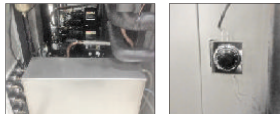
Figure 4-7 Humidifier DI Water Tank & Safety Thermostat
