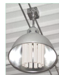
Pan Deck Box Mounting with Hands-Free Hanger
